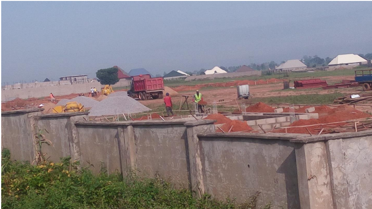
Figure 4.4: Construction of a Boarding Science Secondary School in the study area
