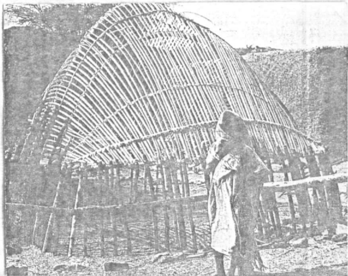
© The making of one unit. (Kraal) sticks being assembled for framework. Skin/hide is later laid on this skeletal structure.
