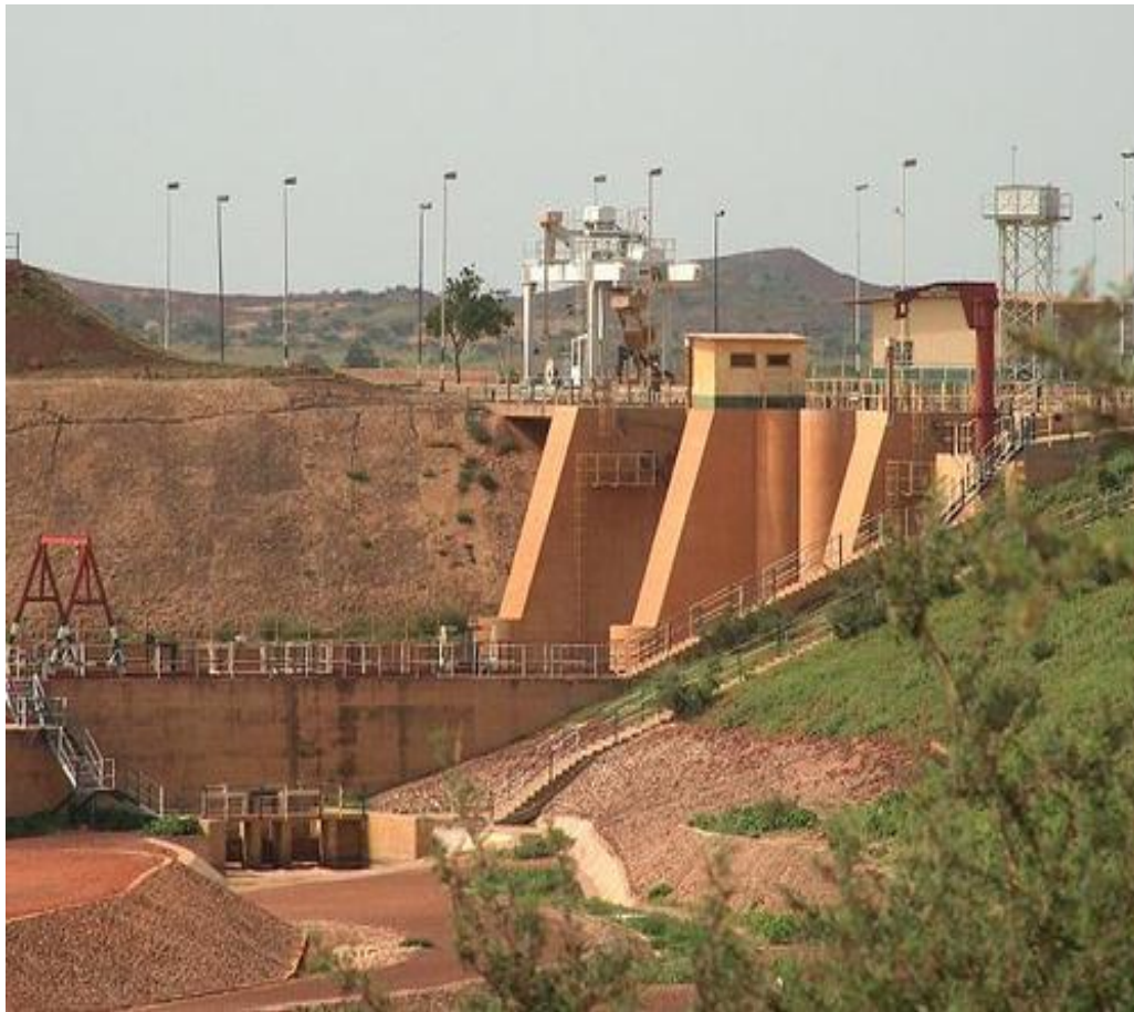
Figure 3.2. Uncompleted structure of Goronyo Dam Source: SRRBRDA, 1991
