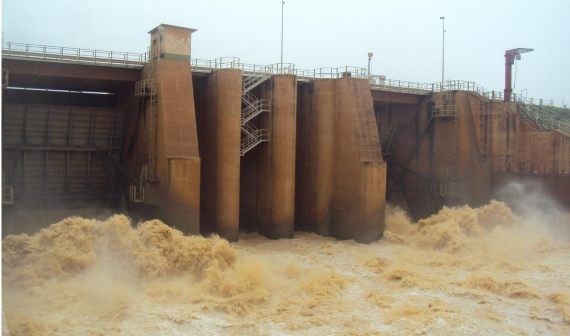
Figure 3.5. Downstream face of Goronyo Dam Source: SRRBRDA, 1991
