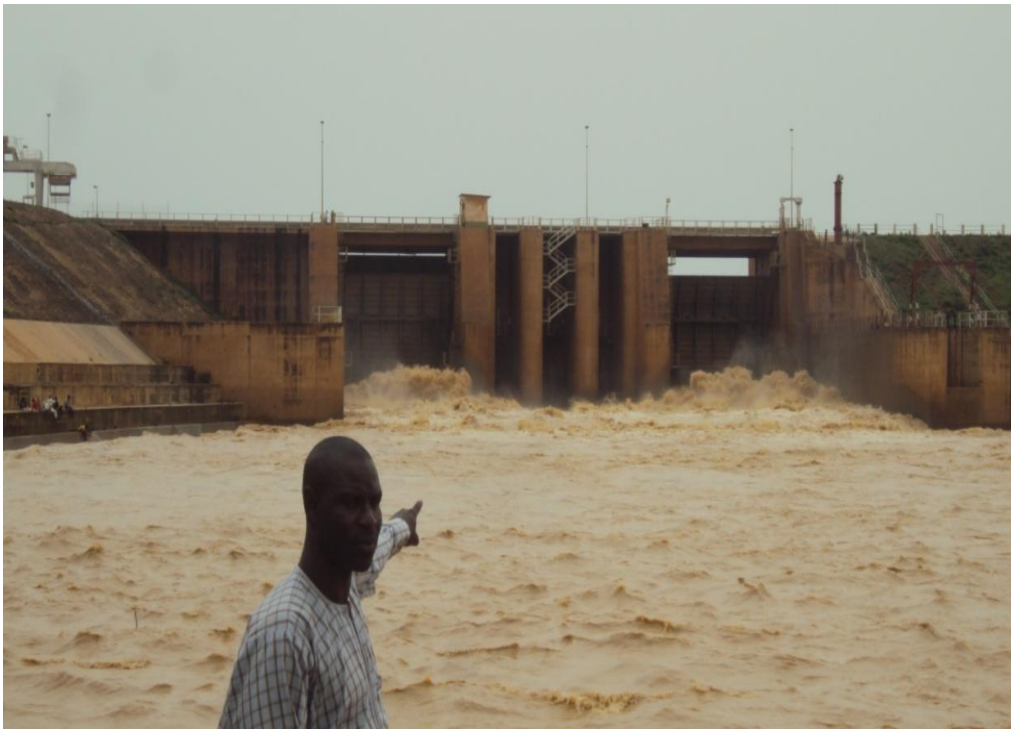
Figure 3.4.Upstream face of Goronyo Dam Source: SRRBRDA, 1991
