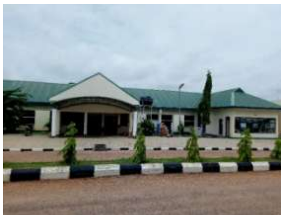
Plate VI: Exterior view of the KASU Library
