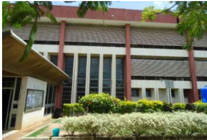
Plate XXVI: Exterior view of Kashim Ibrahim Library shading devices applied
