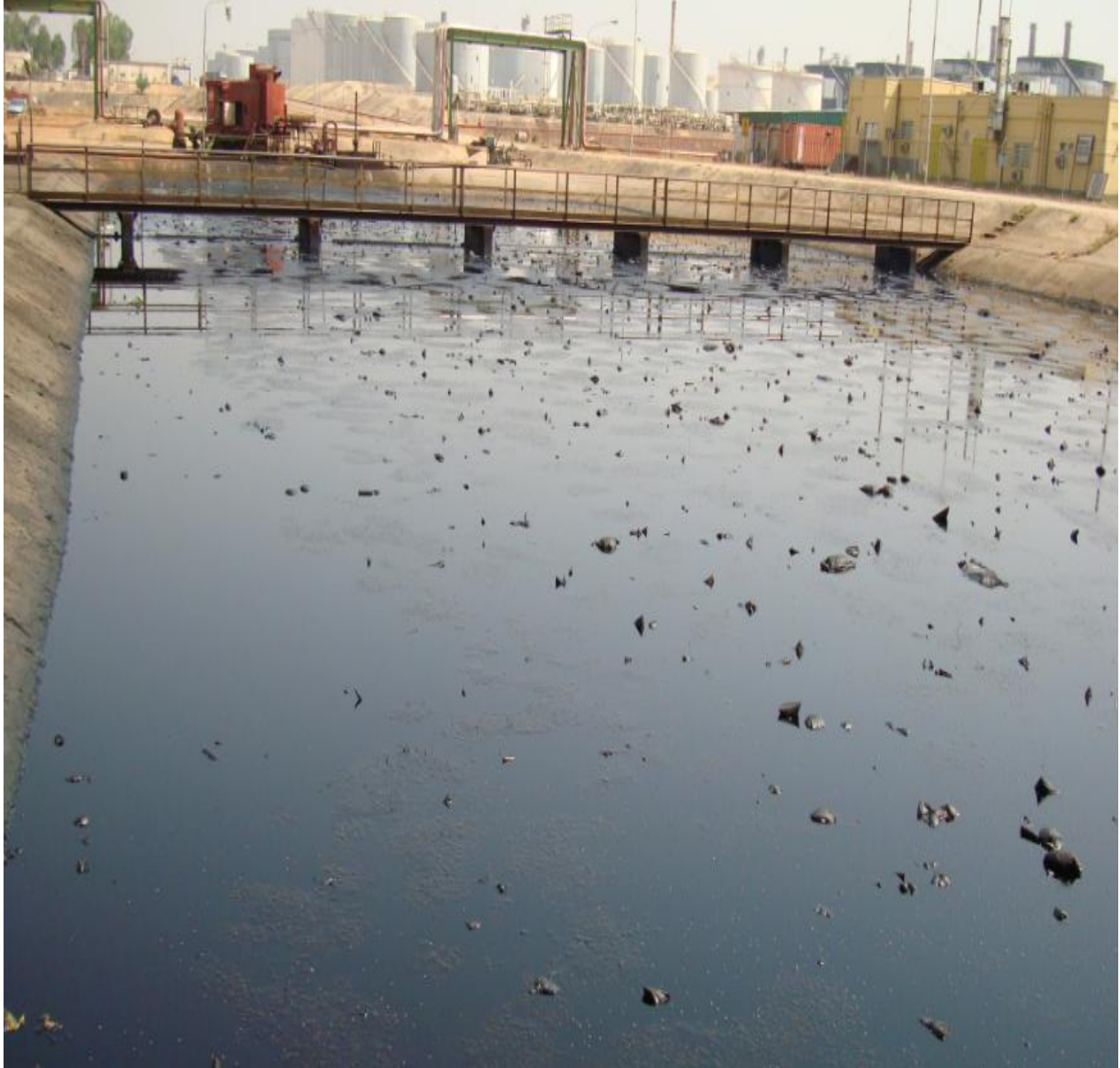
Plate 3b: Waste water Reservoir of the Kaduna Refinery and Petrochemical Company
