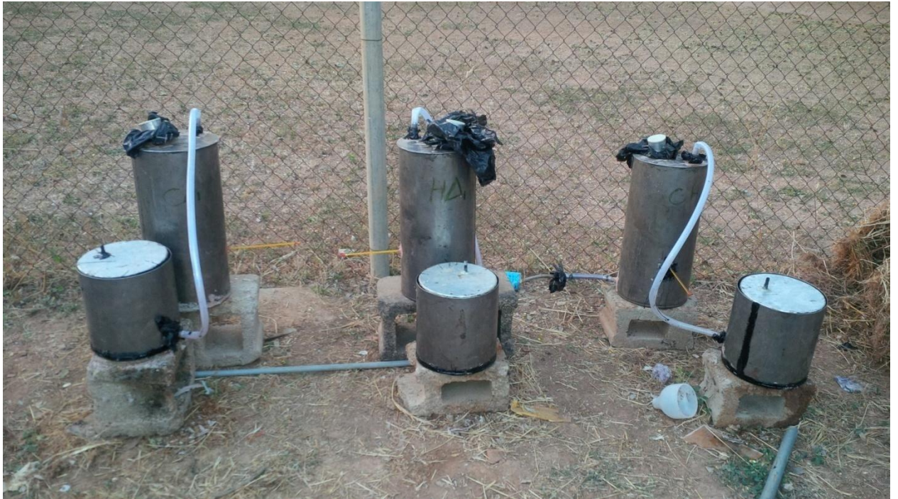
Plate 1: First day step up plant for biogas production.
