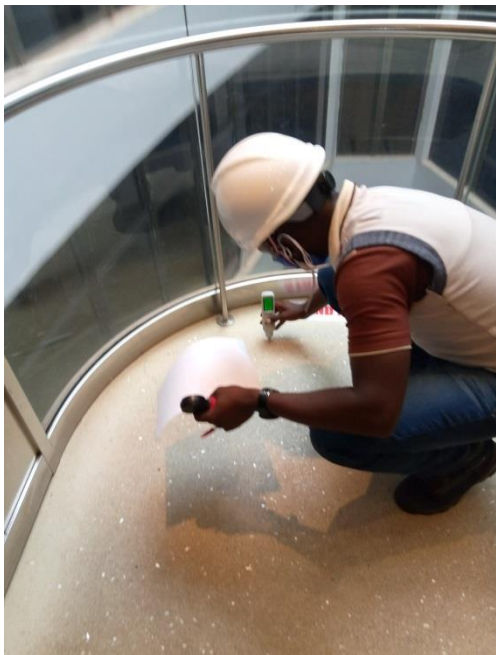
Vibration measurement in panoramic lift car floor
