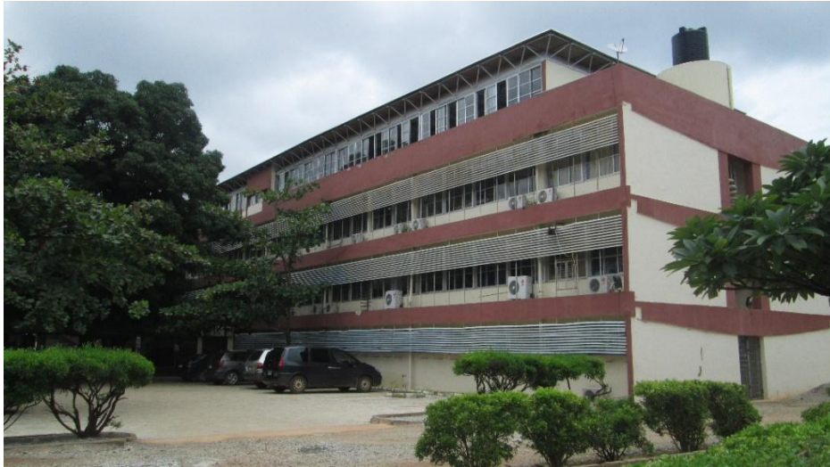
Platexii horizontal shading devices and side-openings Department of Architecture, A.B.U, Zaria.
