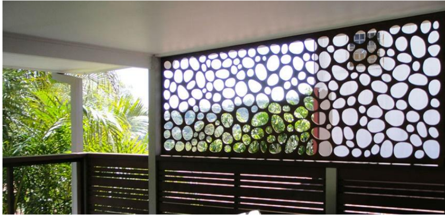
Figure 2.5 Typical Laser Cut Panel System.
