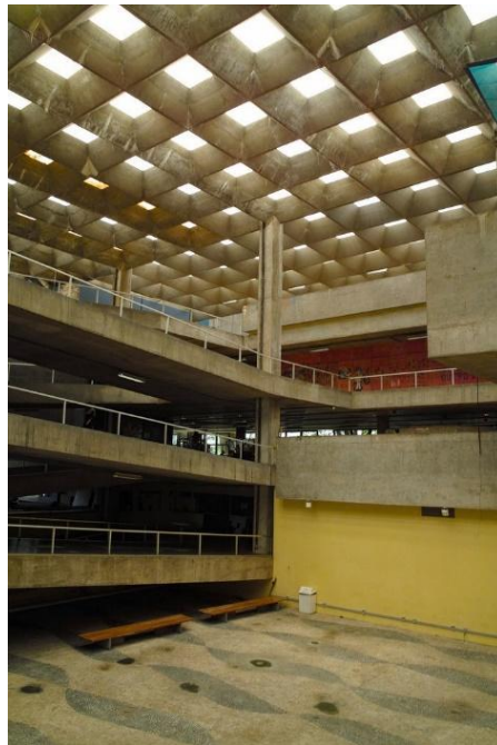
PlatexxTop lighting Faculty of Architecture, University of Sao Paulo.
