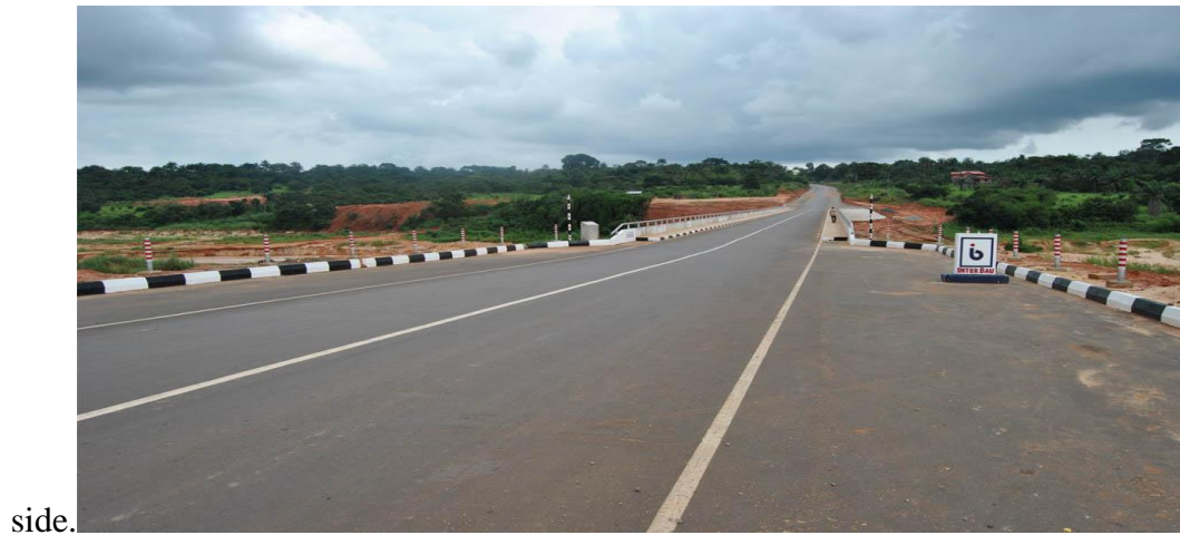
Plate 2.1 Kerb, Along Kaduna-Zaria Road
