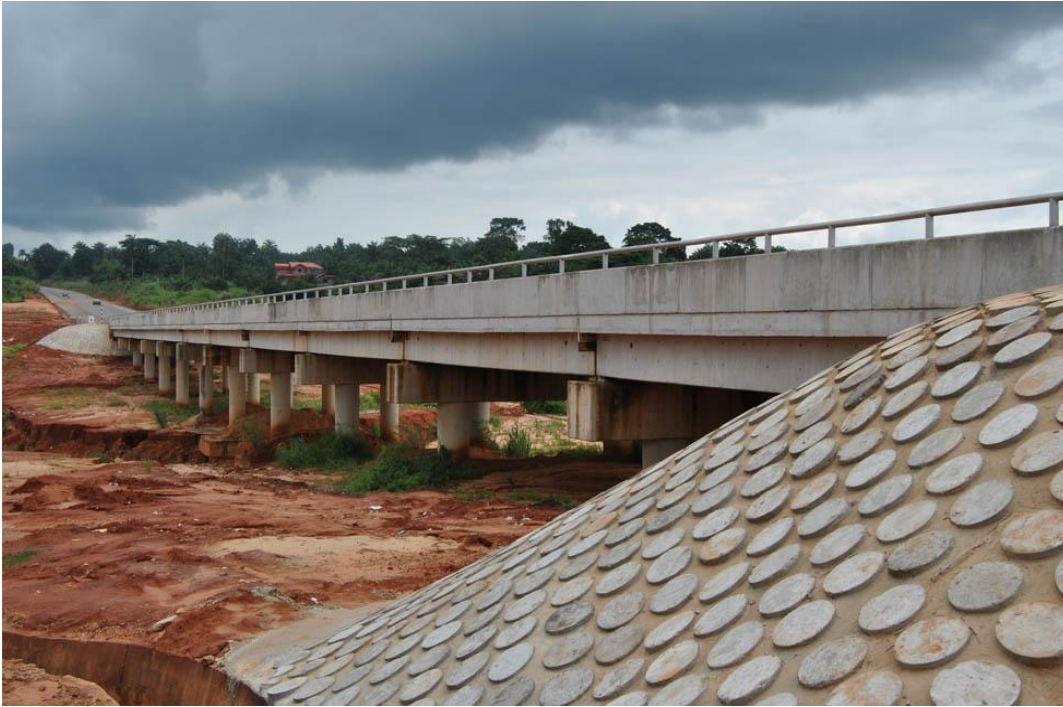
Plate 2.10 Bridge: Kaduna-Kagarko Road (A124) Source: Authors Field Survey (2016).
