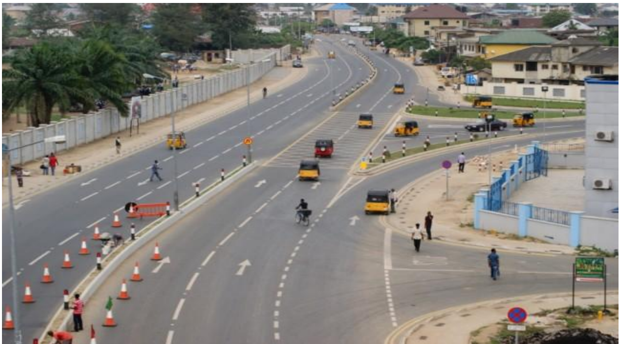
Plate 2.5 Road Marking: Kaduna Town.
