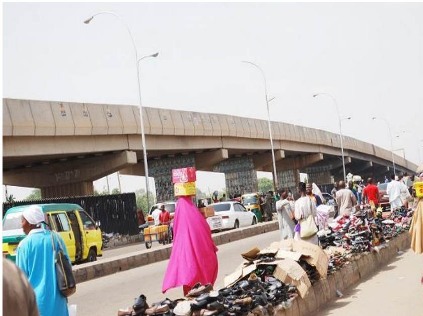
Plate 2.12 Overhead Bridge: Kawo, Kaduna.
