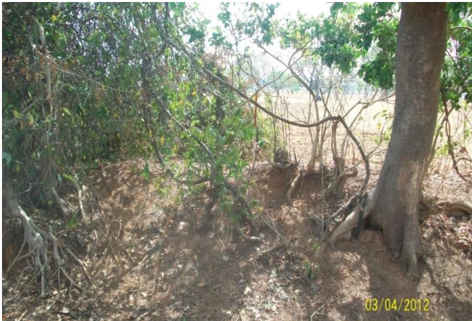
Plate XVIII: Collapsed defensive wall at Tsohon Shado site.
