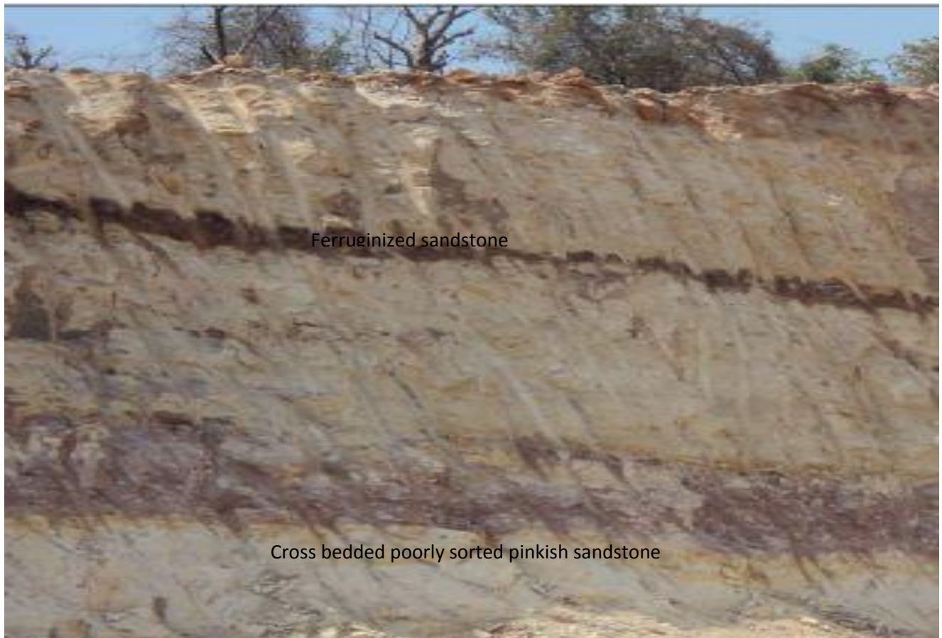
PlateIII:Road section of the Lokoja Sandstone showing feldspathic poorly sorted cross bedded sandstone at km 4.5 along Lokoja-Abuja express way.(7°51'54.9"N and 6°47'29.6"E)
