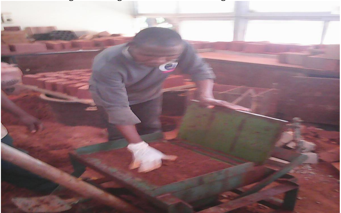
Plate VI Moulding of Bricks
