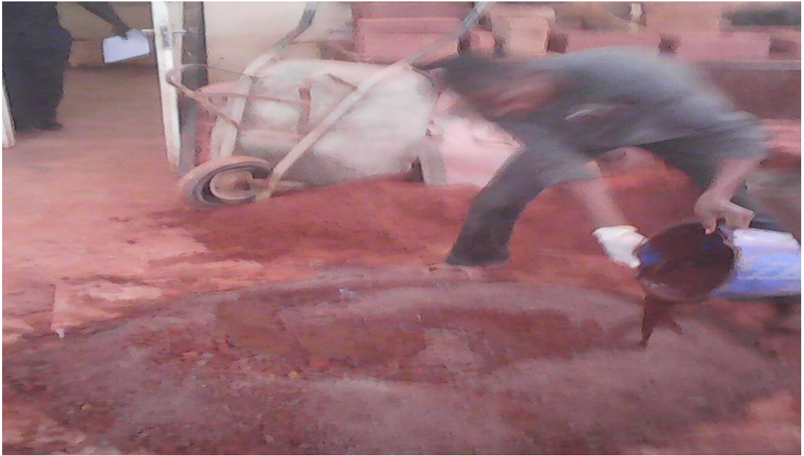
Plate V Batching and mixing of laterite with 3 binding media
