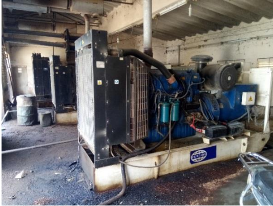
Plate III: 2300KV Generator serving as power alternative
