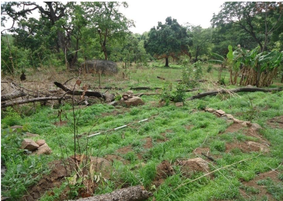
Plate XXvii: House Foundation at Awai (Photographed by Sankyai Obadiah, 2013)
