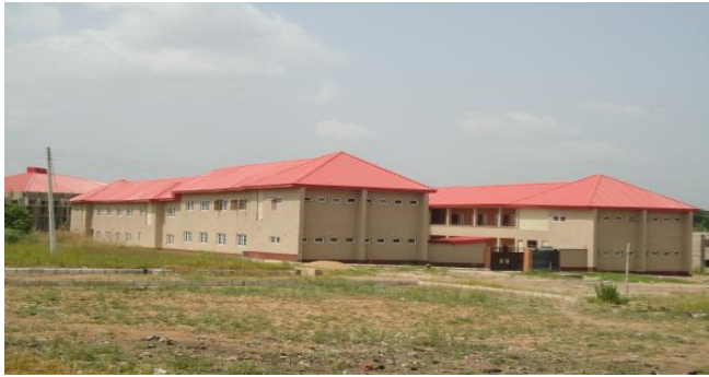
Plate 4.5 A newly Constructed Female Hostel in BSU by TETFUND
