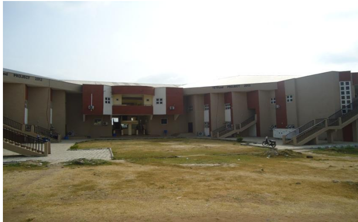
Plate 4.8 Twin Lecture theatre constructed by TETFUND in BSU
