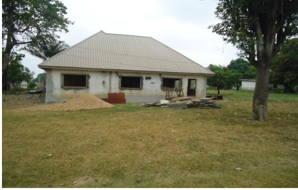
Plate 4.11 A Staff House Undergoing Renovation in BSU
