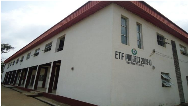
Plate 4.2 A Renovated Laboratory in BSU by TETFUND
