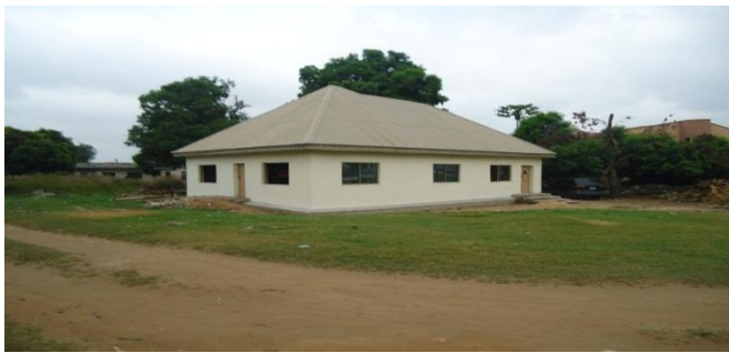
Plate 4.10 A Recently Renovated Staff House in BSU
