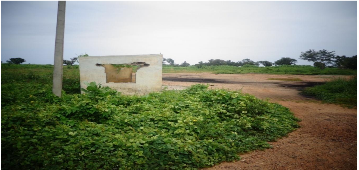
Figure 4.6: Dilapidated building said to have been dumped by workers on the road
