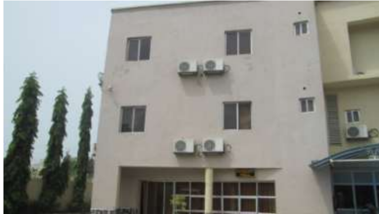
Plate XI: Exposed windows and walls of the Jamil hotel, Bauchi.
