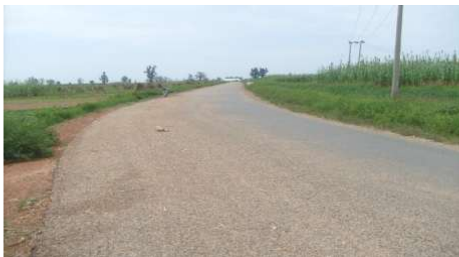
Plate II: Trunk C Road Doka-Likoro road
