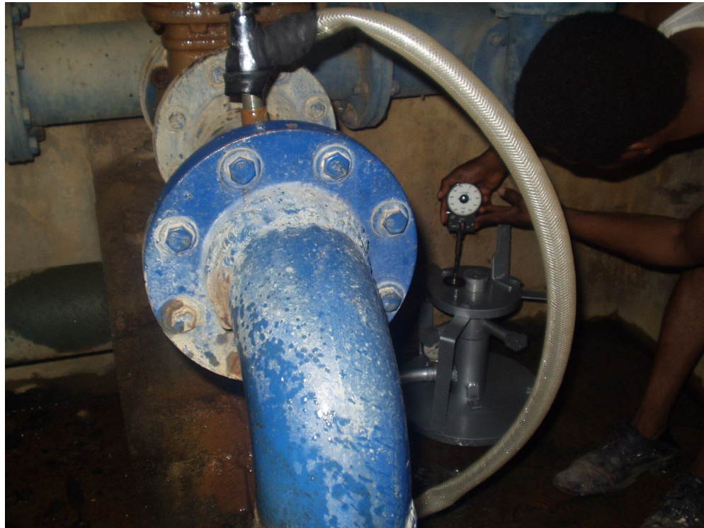
Plate IV: Measuring Speed and Pressure under no Load Condition
