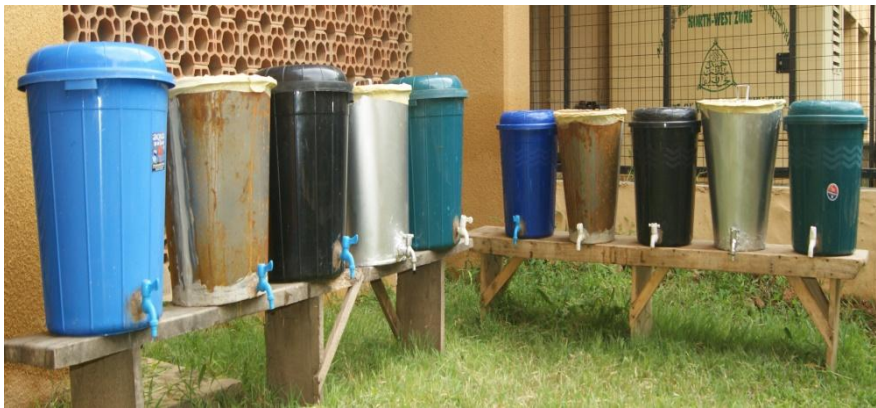
Plate 3.2a: Water storage containers installed outdoor (for both borehole water and tap water).
