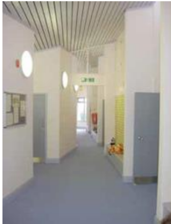
Plate I: The use of noise and echo treatment for floor and ceiling –Source: Torkey (2013)
