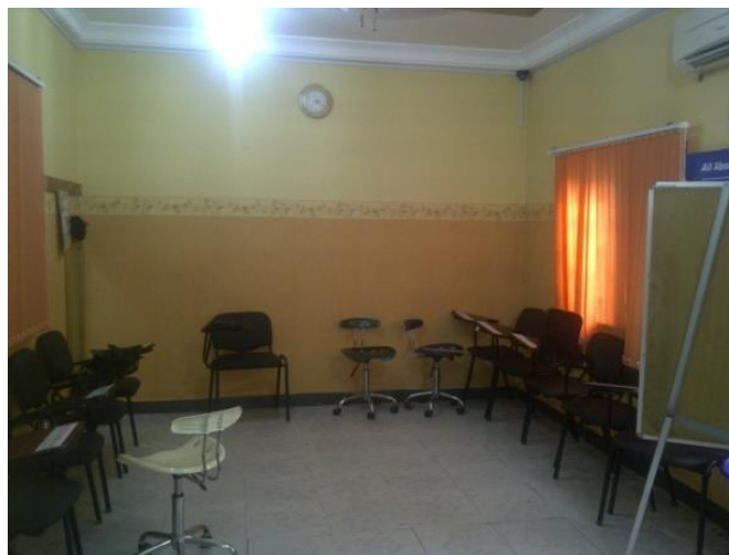
Plate XXII: Terrazzo floor finish and POP ceiling in Group class
