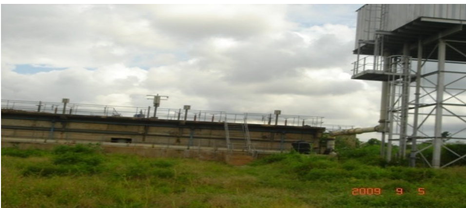
Plate 5.3 show part of the treatment plant
