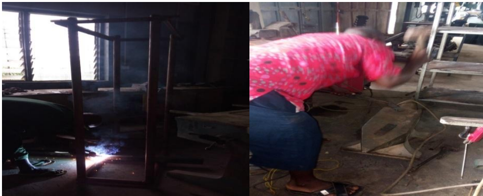
Plate III: Welding of the rail track
