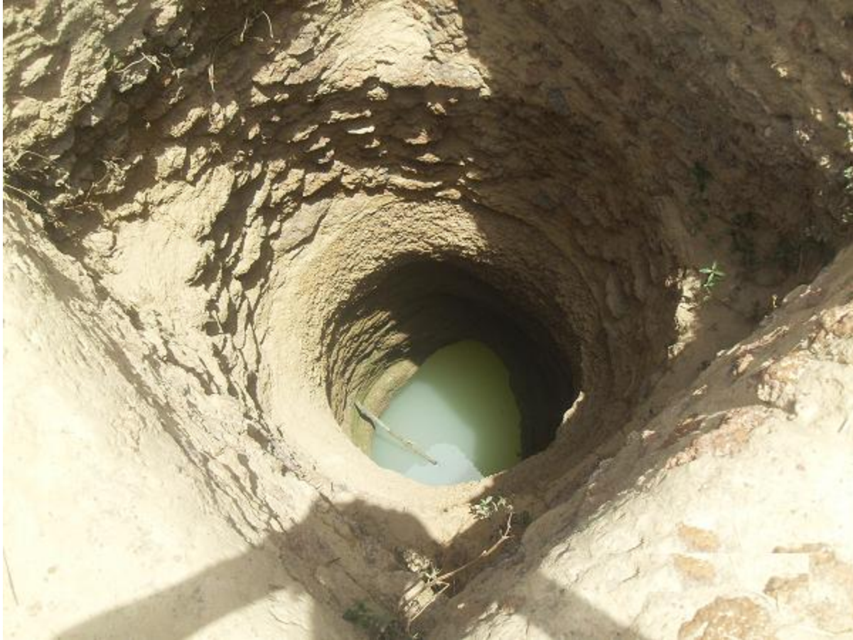
Plate 1: An unprotected hand-dug- a well major source of water in Damuga and other communities before the MDGs intervention Source: Field survey, 2013
