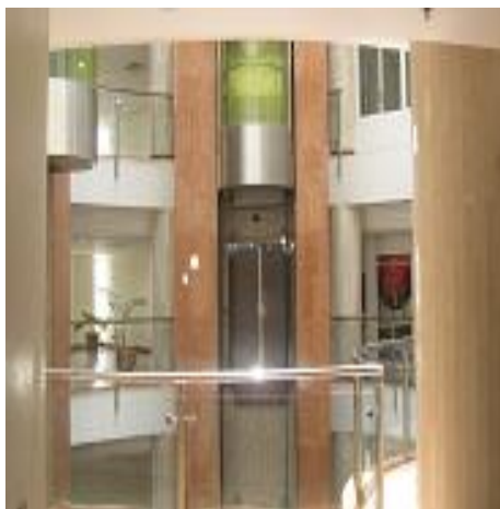
Plate 4.7: Views of lift openings Source: Researchers work, 2014.
