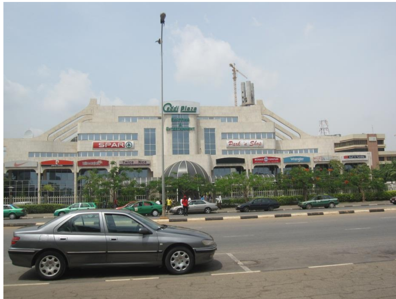
Plate 4.1: External view of Ceddi plaza Source: Researchers work, 2014.
