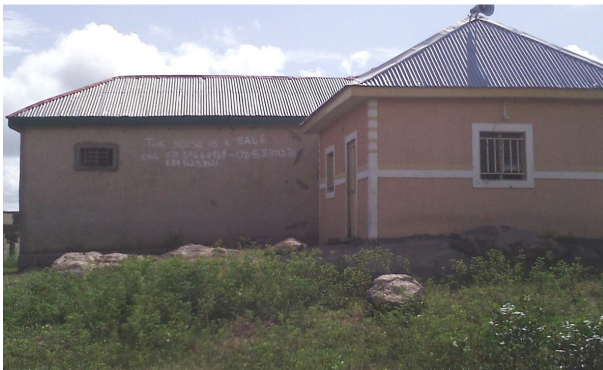
Plate ix: Poor location of building. (Source field survey 2015).
