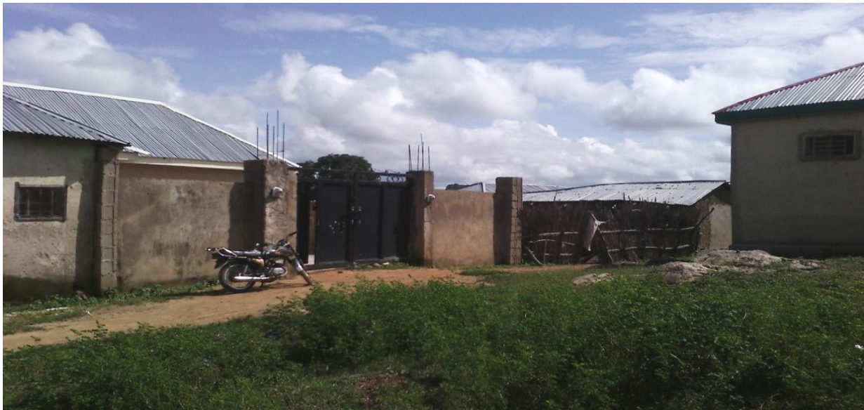
Plate xiii: Housing condition in Bauchi town. (Source field survey 2015).
