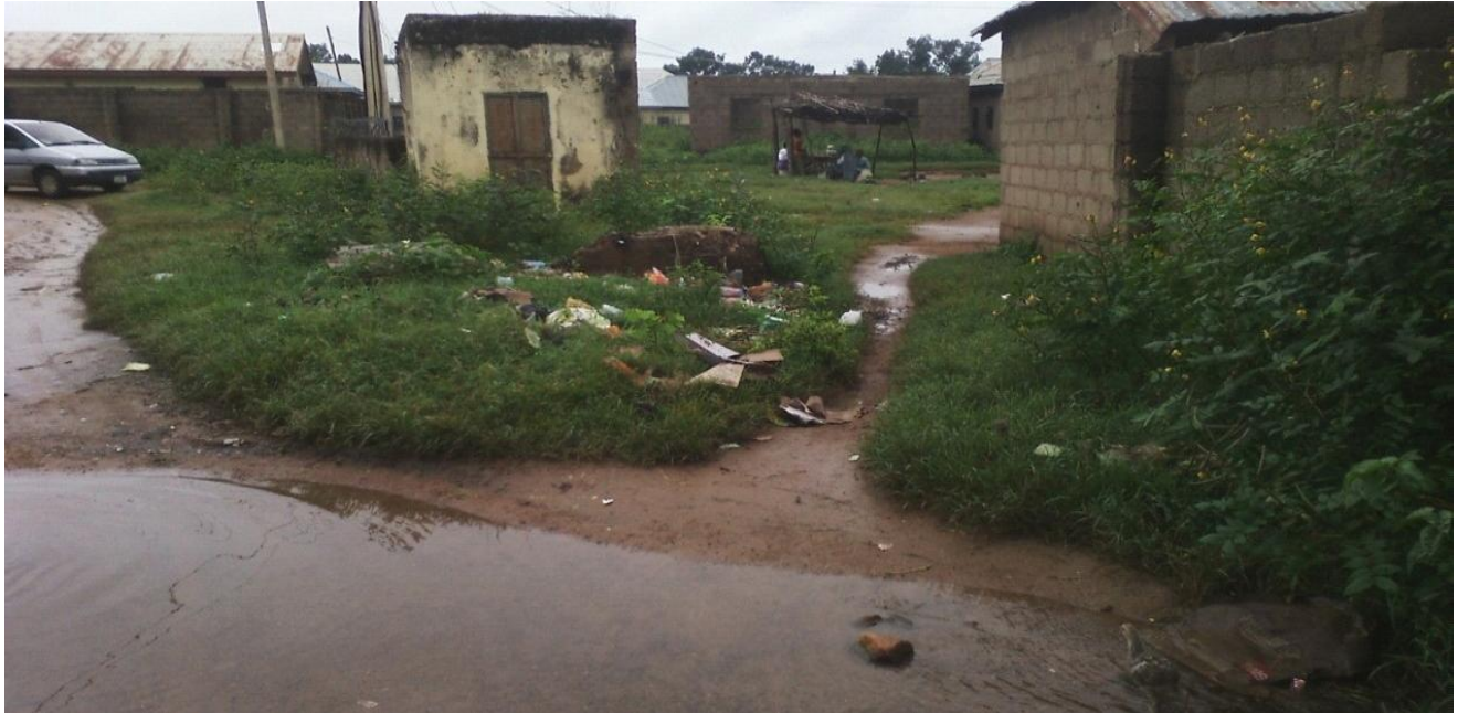
Plate .xii. Poor road network without drainage.(Source field survey 2015).
