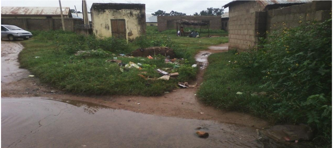
Plate .iii. Poor road network without drainage. (Source field survey 2015).
