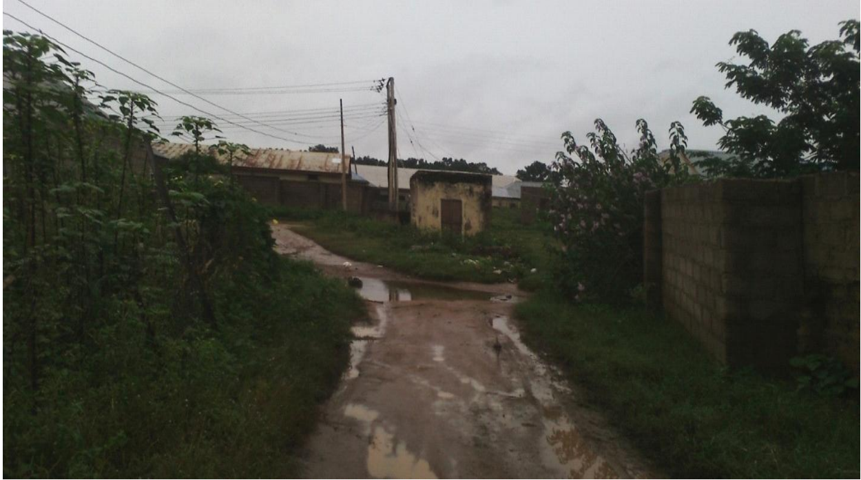
Plat iv. Poor road without drainage (source field survey 2015).
