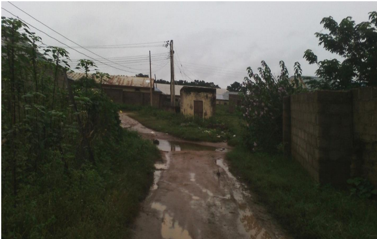
Plate vi: poor road, electric supply and drainage. (Source field survey 2015)
