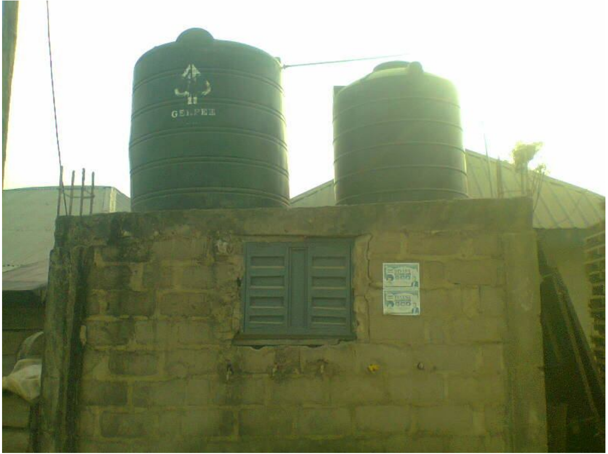
Figure 3.4 Picture of a borehole in site 2 (Obajana 8)
