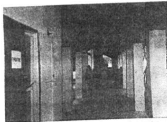
Plate 5-12 Covered walkway between theatre and Leprosy ward
