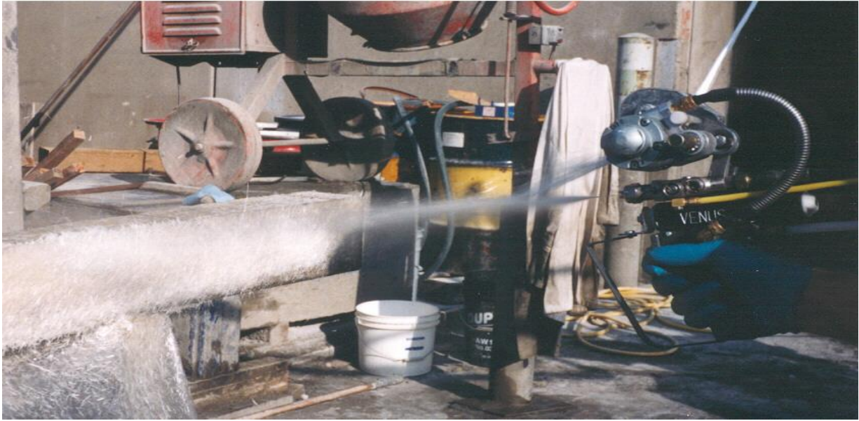
Plate 1: The Spray Operation
