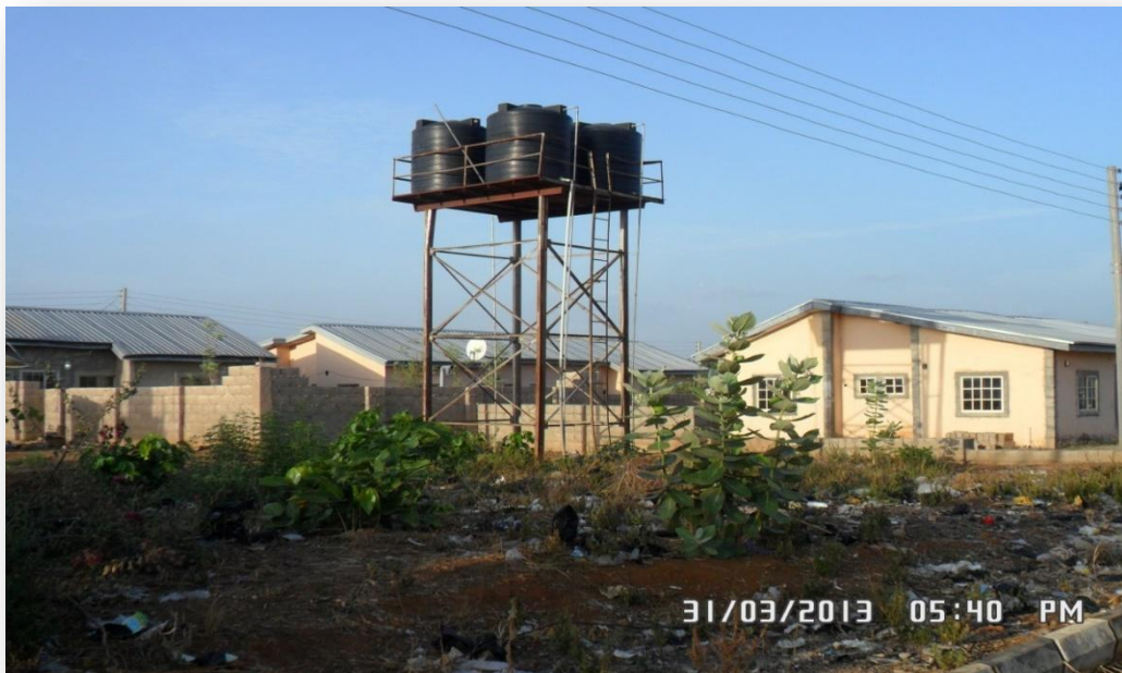
Plate VIII: Constructed drainage and culvert by Bosso Estate Development Association
