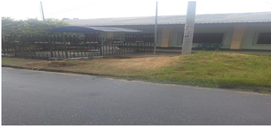
Otusega Community Hall where the TFD intervention at Otusega was done
