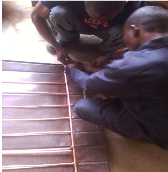
Plate 1: Construction of copper grid
