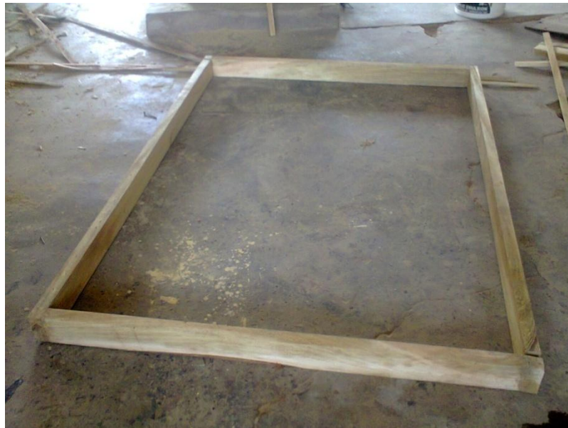
Plate 2: Construction of collector casing from dry wood
