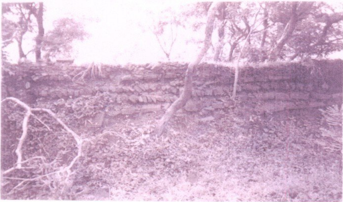
Plate 13: The walls strengthened by slabs at old Birnin Gwari
