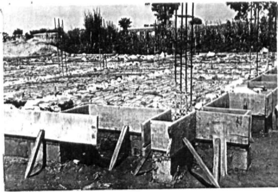
Figure 4a: Hardcore filling completed with uneven spread of wire mesh
