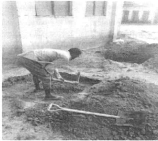
Plate 1: Pits to access the foundation
