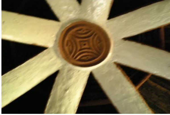
Plate 4.2.6: Rib structural beams joint.
