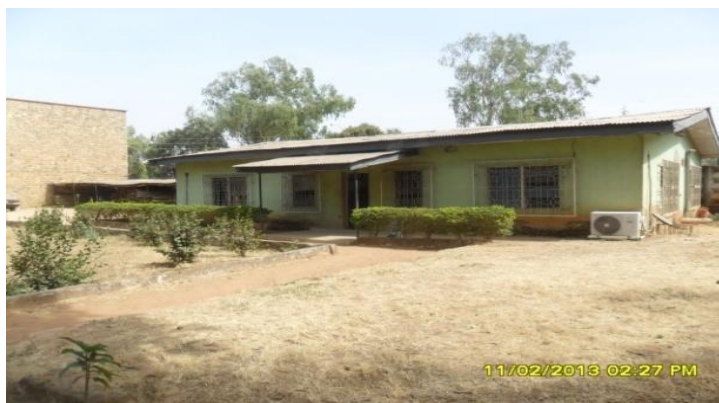
Plate 4.3: Approach view of the administrative block.
