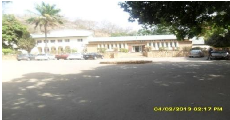
Plate 4.3.2: Approach view of the main gallery.
