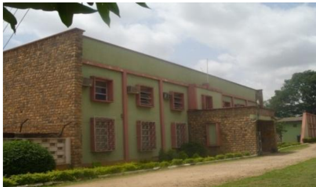
Plate 4.2: Approach view of the main gallery.
