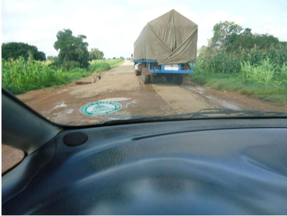
Plate 4.3: Hotspot Location with Potholes/Eroded Shoulder along Birinin Gwari Road Source: Field Survey, 2016
