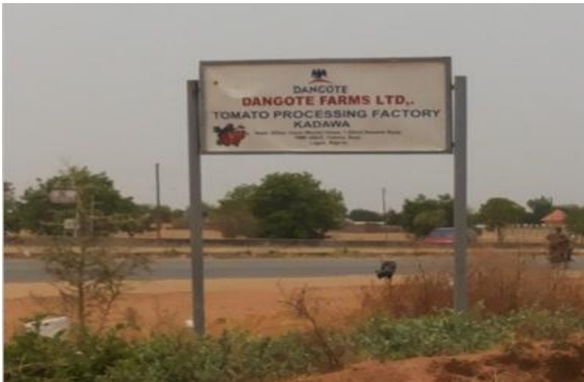
Plate 5: Dangote tomato processing industry under construction in the study areas
