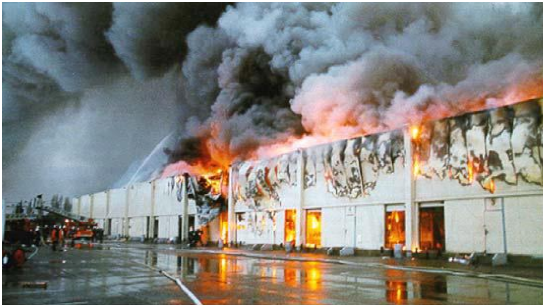
Plate IV: The intense heat radiation of a fire forces the fire services to keep their distance from
