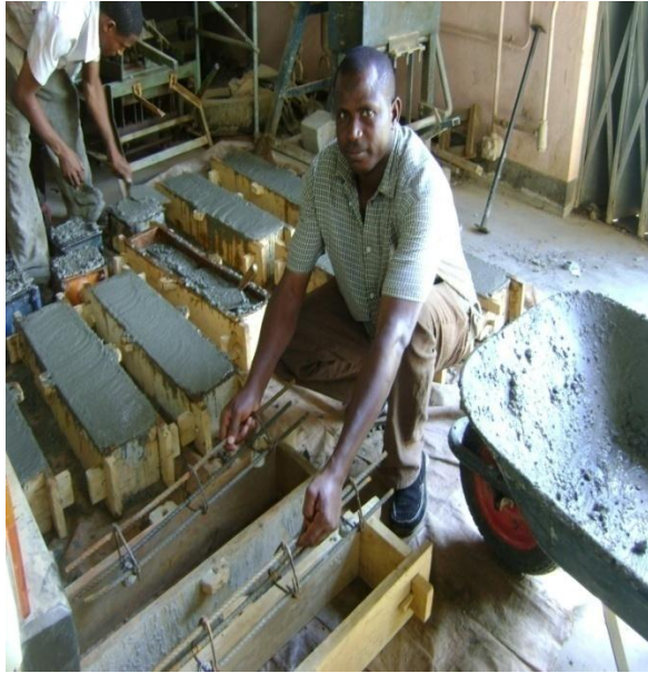
Appendix A-7: Casting of specimens in progress
