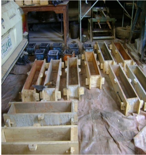
Appendix A-6: Setting of moulds for casting
