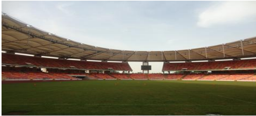
Plate I: Side view of the Main bowl of the COJA sporting facility in the Federal Capital City Abuja (Source: Author's Field Survey, 2015)
