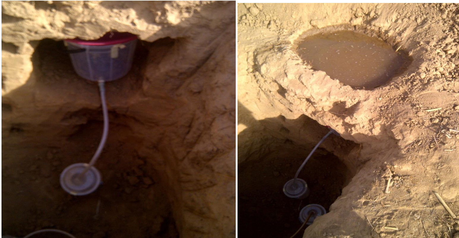
Plate 3.3: Free drainage lysimeter installation in the field
