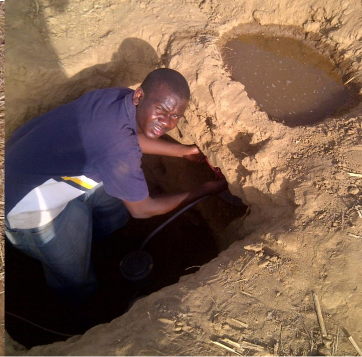
Plate 3.2: Scientist installing free drainage lysimeter in the field
