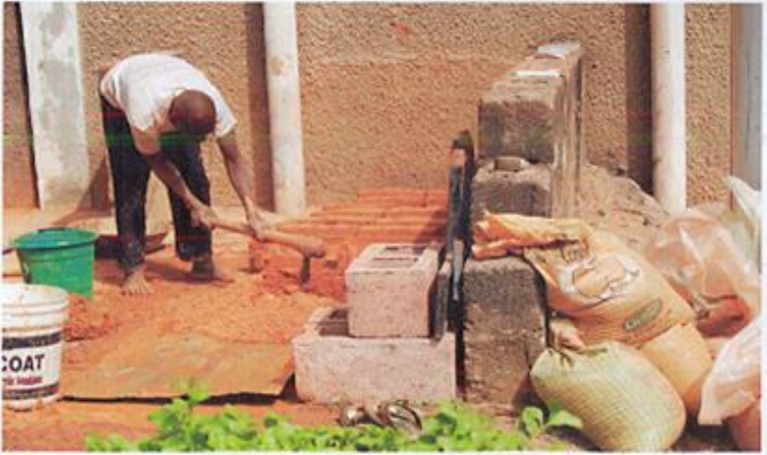
Plate 4: Wetting of soil and moulding blocks
