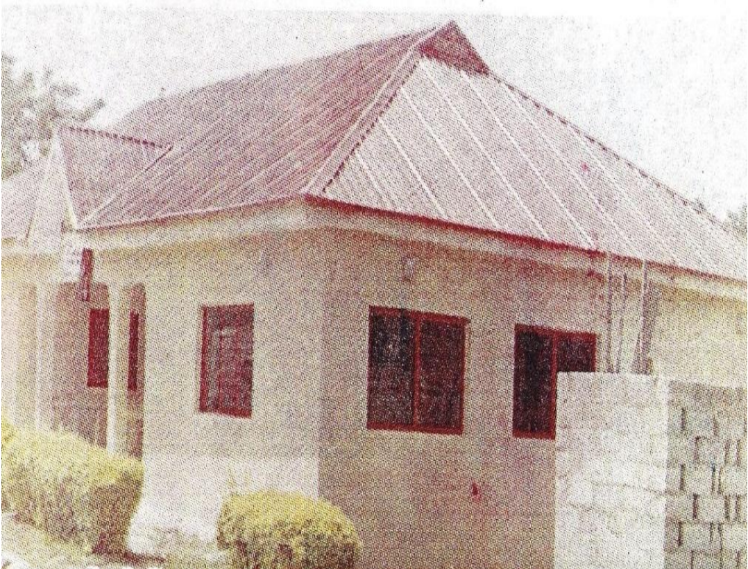
Administrative Complex Built by the Underprivileged Lots Concern Group for a Neighbourhood School in Mararaba
