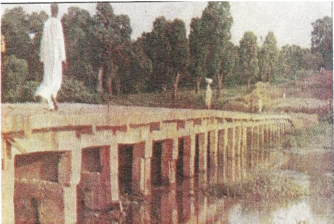
Umaisha-Zineku Bridge Constructed by Toto Local Government Progressive Union in Umaisha, 2012/2013.
