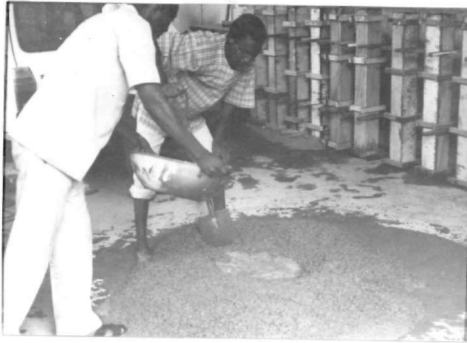
PLATE 5: MANUAL (HAND) MIX OF THE CONCRETE USED FOR THE CASTING
