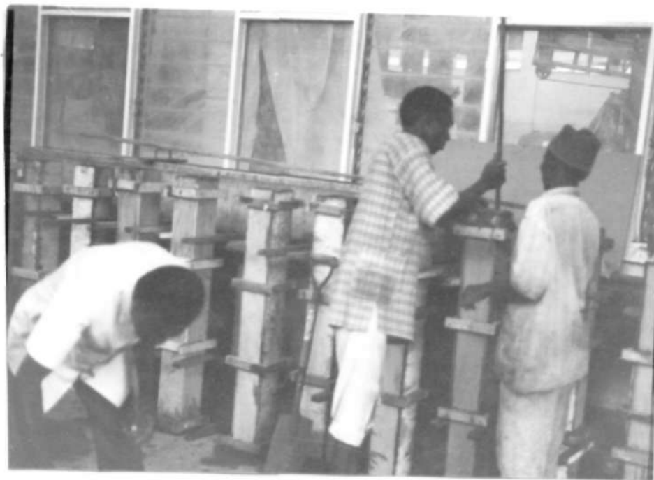
PLATE 6: THE RODDING METHOD OF - COMPACTION USED DURING THE CASTING
