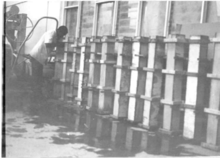
PLATE 3: ARRANGING OF THE FORM WORK IN READINESS FOR THE CASTING
