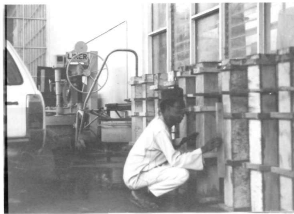
PLATE 4: PLUMBING OF THE FORM WORK TO MAKE SURE THE COLUMNS ARE CASTED VERTICALLY.
