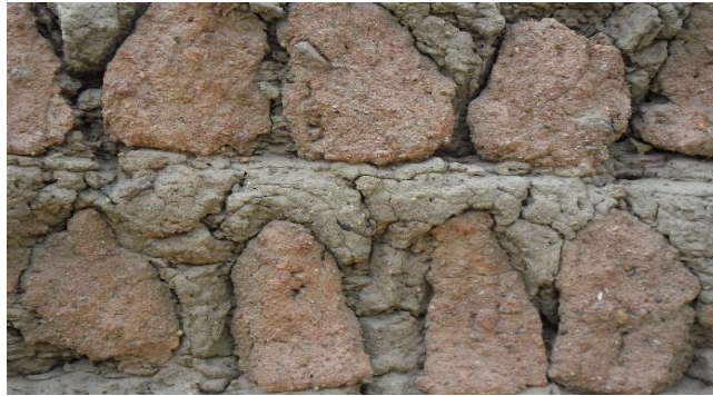
Plate VI: Tubali bonded in mud mortar
