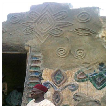
Plate VII: Makuba stabilised mud rendered wall in Zaria city
