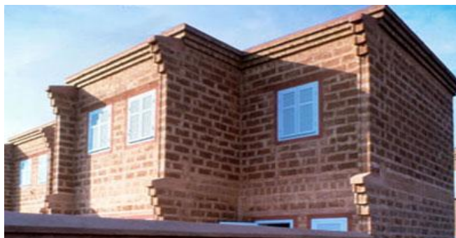
Plate II: Compressed Earth Brick Storey Building
