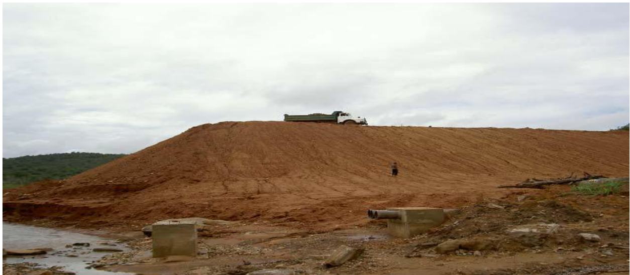
Plate 3.2: Part of the Quarry site
