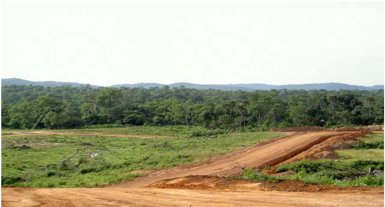
Plate 3.6: Road leading to the Quarry site
