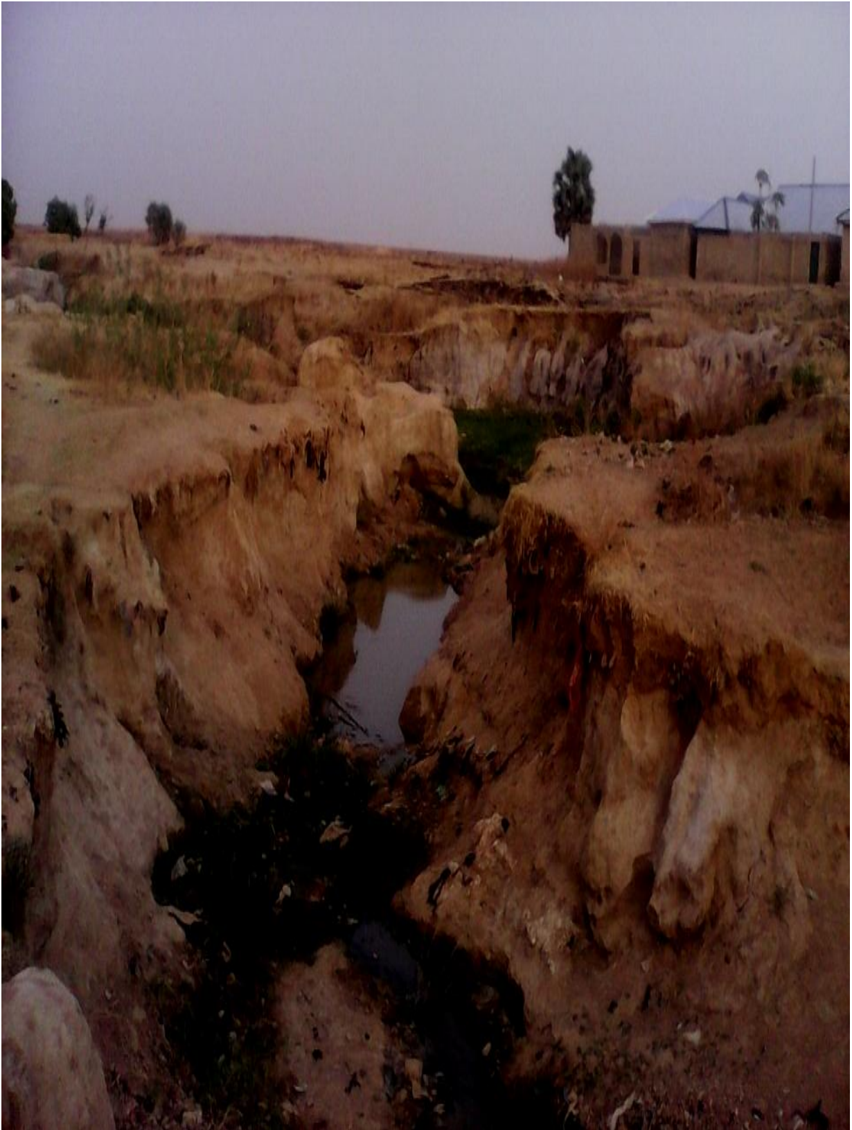
Plate VIII: An overview of severe gully erosion at Ungwan Danyaro.
