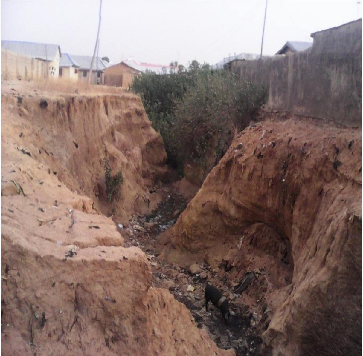
Plate VI: Gully advancing towards building foundation
