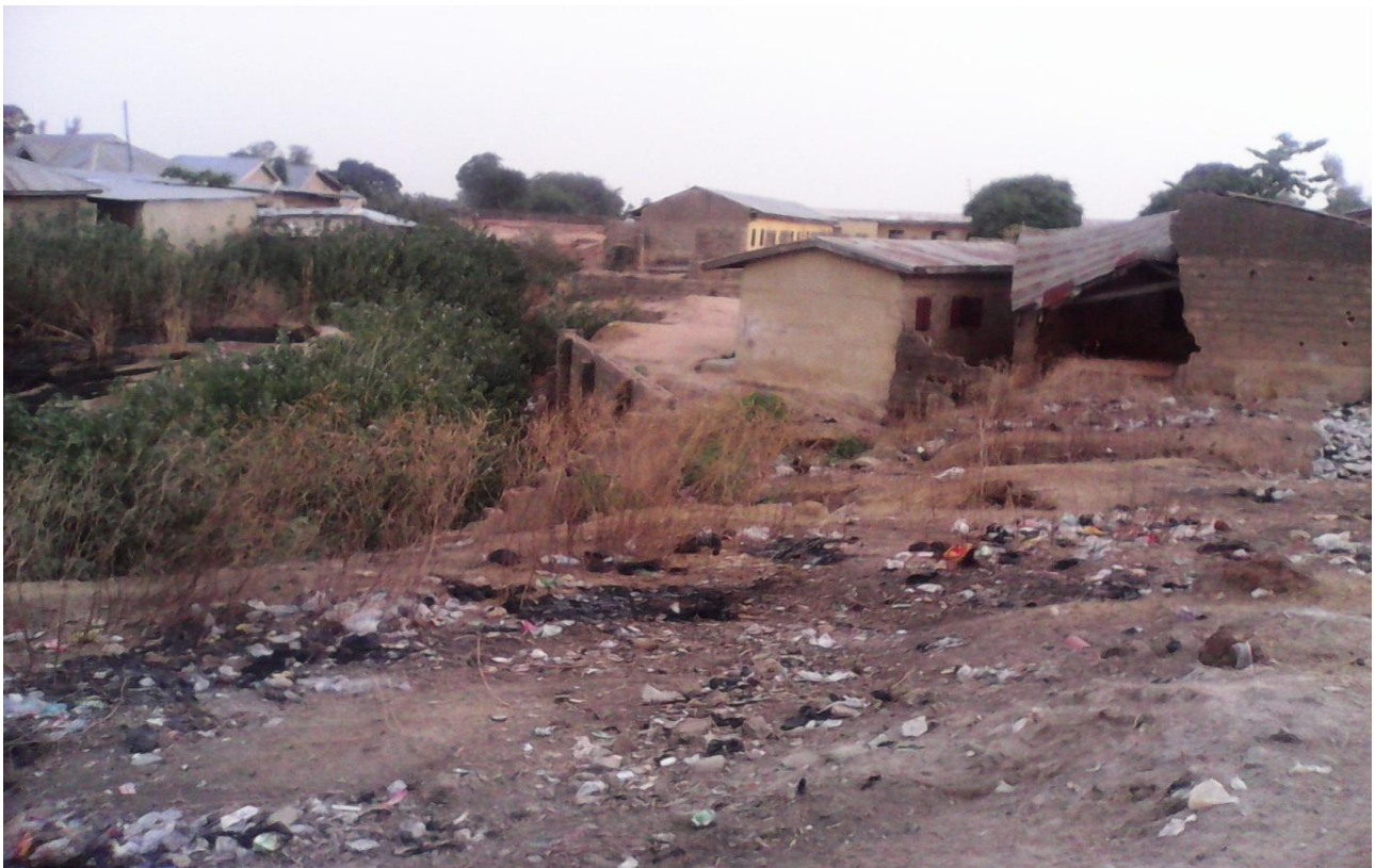
Plate II: God's Time Secondary School buildings collapsed as a result of Gully erosion.
